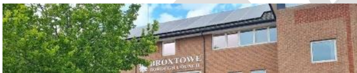
Image 3: Solar PV on the main Council offices at Foster Avenue, Beeston
